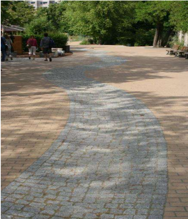
Rainwater drains along this channel
