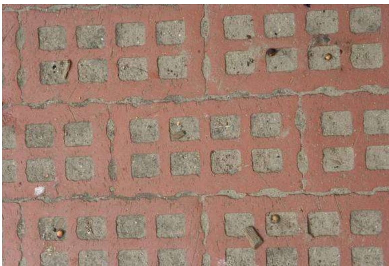
Common surface type. Sandy soil in holes - with weeds growing in areas of lower use
