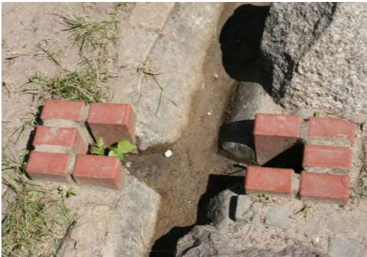
...with sluice gates
