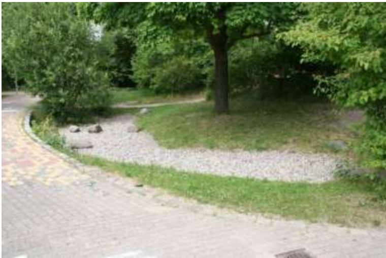
Rainwater from the higher part of the playground drains into this play splash pool
